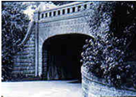
LAKE ALVORD BRIDGE
